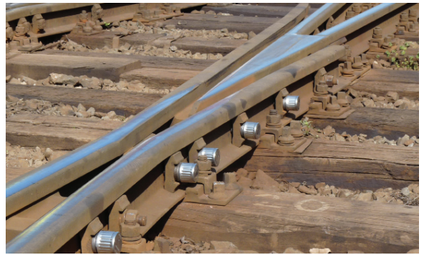
Hungarian state railway MÁV is using Tracksure fastenings to secure turnout crossings.
